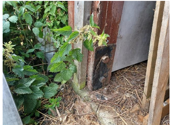
Photo 2: Structure comprising timber frame with corrugated asbestos cement sheet cladding, asbestos verge caps and cladding angles.
