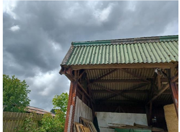
Photo 2: Structure comprising timber frame with corrugated asbestos cement sheet cladding, asbestos verge caps and cladding angles.
