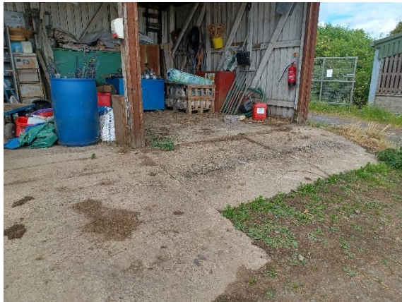
Photo 9: Entrance to LHS of shed, concrete slab in fair condition with localised deterioration.
