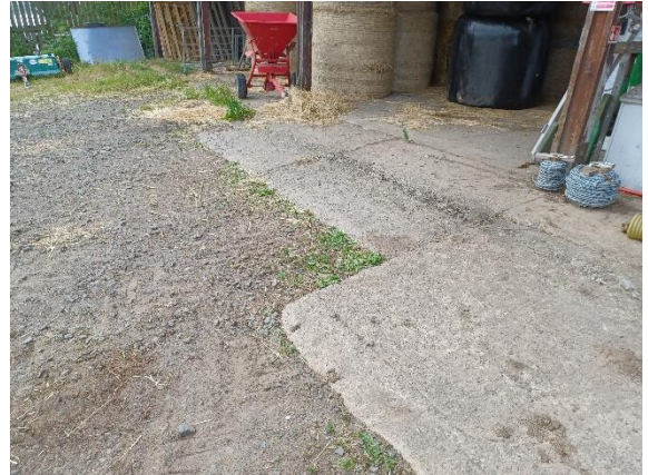
Photo 8: Entrance to LHS of shed, concrete slab in fair condition with localised deterioration.
