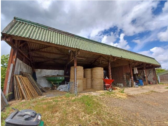
Photo 1: General view of principal elevation
