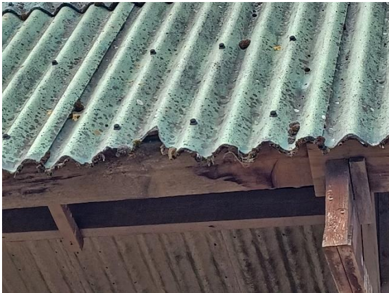
Photo 3: One of several damaged asbestos sheets at leading edge of canopy.
