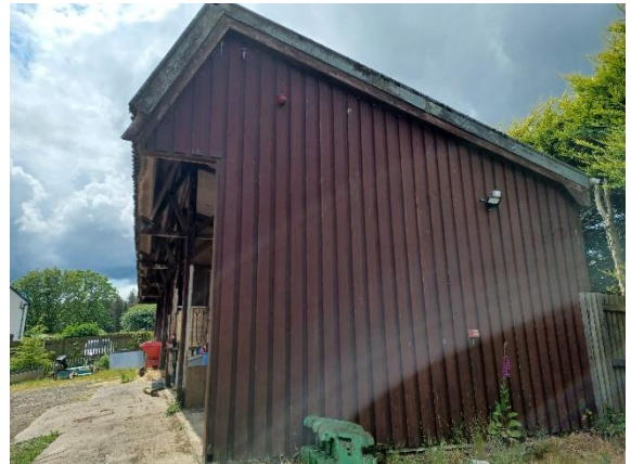
Photo 8: Entrance to LHS of shed, concrete slab in fair condition with localised deterioration.
