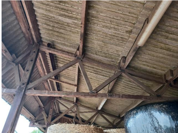
Photo 7: General view of underside of roof.
