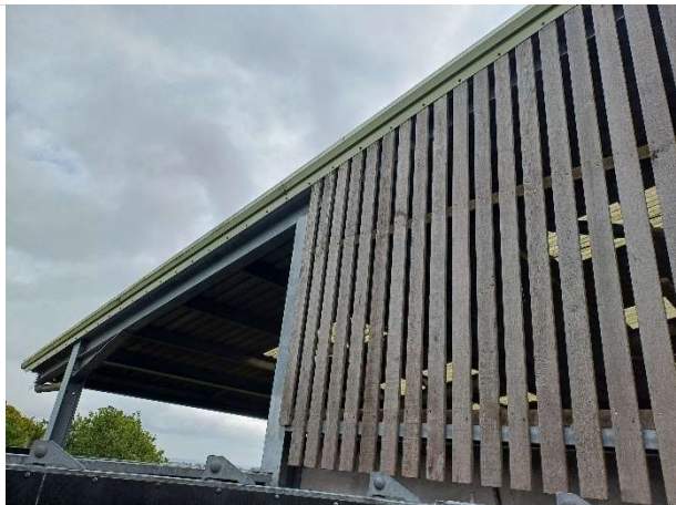
04 Wooden cladding on left elevation in satisfactory condition.
