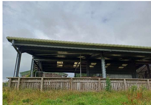
05 General view of rear elevation.
