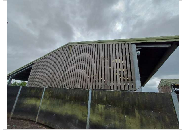
03 General view of left elevation.
