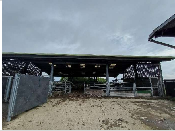
01 General view of front elevation.
